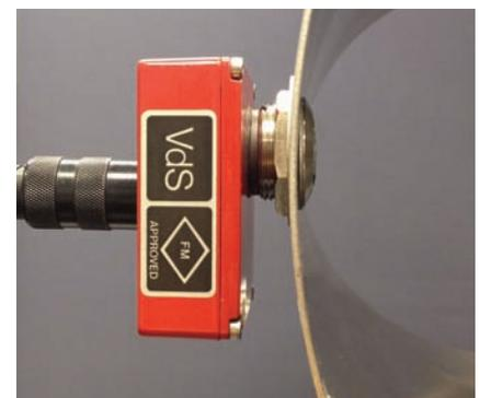
Figure 4. IR spark detection mounted flush on duct wall with as little protrusion as possible using stainless steel adapters. The label indicates this spark detector is Factory Mutual approved.
